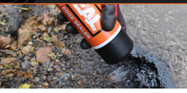
BituSeal is a premium performance aerosol edge sealant; the formulation includes a high concentration of flexible bitumens for ultimate long lasting results.
