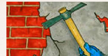
2. Remove the damaged plaster to about 1 meter above the affected areas. Remove all loose materials. Replace crumbly or degraded bricks.
