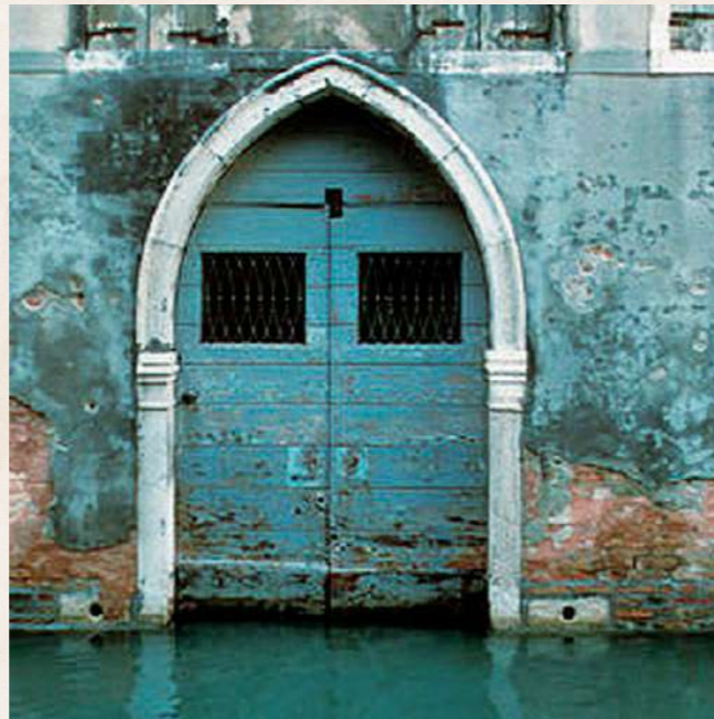
Typical application example of the Rinzafo MGN lime plaster in Venice: degraded, salty masonry in direct contact with water
