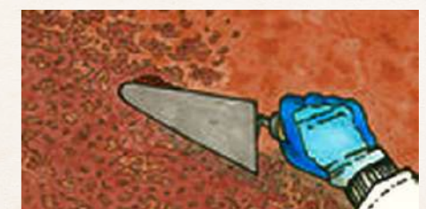
6. Allow the RINZAFFO MGN scratch coat to dry. For wet areas repeat the process.
