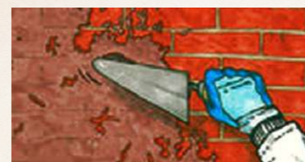
4. After the surface has been adequately wetted apply the RINZAFFO MGN scratch coat onto the entire surface in a 10 mm layer (min 5 mm).
